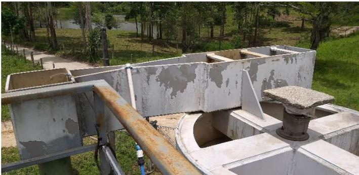
Figura 11: ETA - Calha Parshall.
